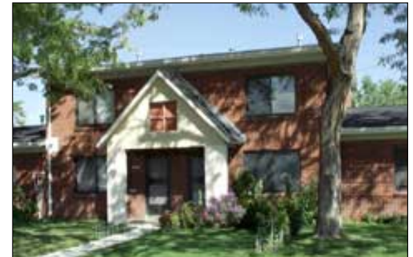
Recently renovated Quigg Newton homes
